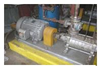
Boiler Feedwater Pump (Controlled by a VFD)
